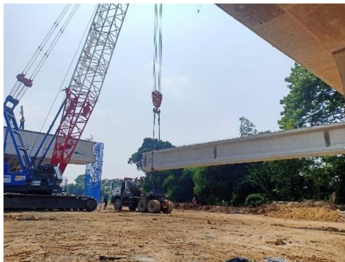
Gambar 1 Proses Erection Girder Sumber: Data Peneliti, 2025
